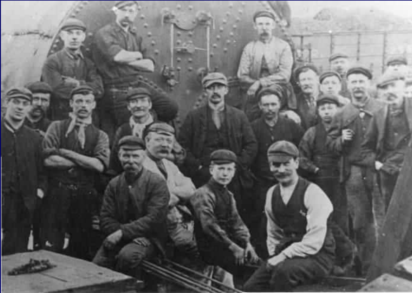
SURFACE WORKERS AT CAMBOIS COLLIERY. BOILER HOUSE HAD A HAND-FIRED BOILER. PHOTO FROM DAVID DURWARD'S COLLECTION
